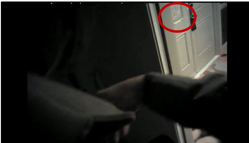
(Bullet holes in door to Room 32-135 prior to breach.)
